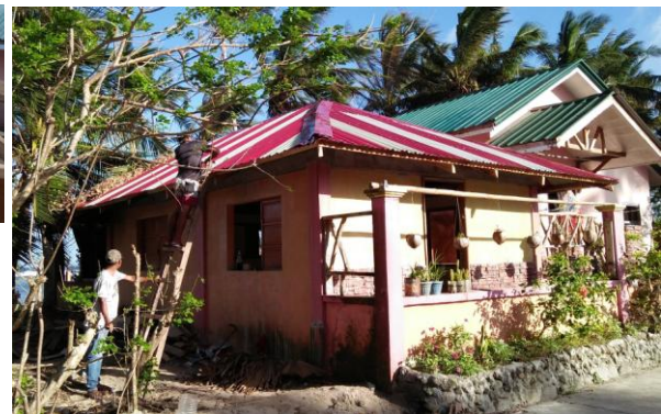
Candumaay Matnog Church before and after reroofing, replacing a woven roof with stronger corrugated steel.
