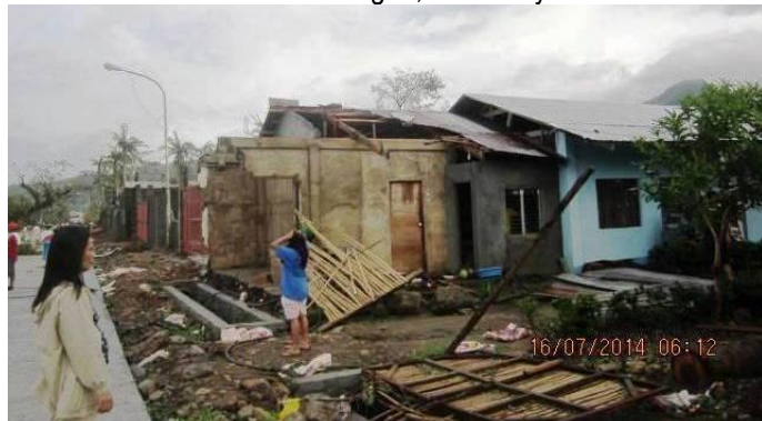
EBI bamboo front fence was blown down and Pastor Raf's house (the former bakery) had roofing blown off.
