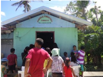
PAMI Fabrica church with roof repaired
