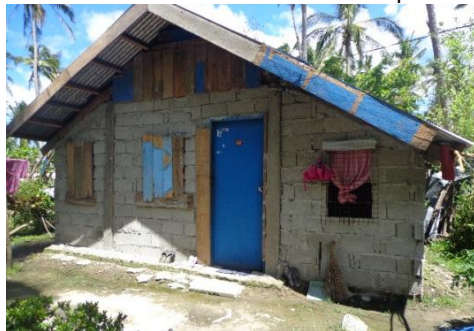
A repaired home in Tanga, Bulan
