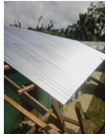
EBI dorms are being refurbished, including new roofing.
