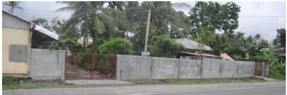
New EBI cement front wall and steel gates (far left is Ptr Raf's house)
